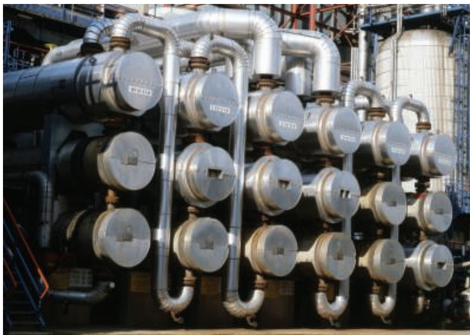
FIGURE 1. Heat exchangers in many CPI applications can experience tube rupture, and these scenarios must be evaluated and addressed in order to ensure continued safe operations
